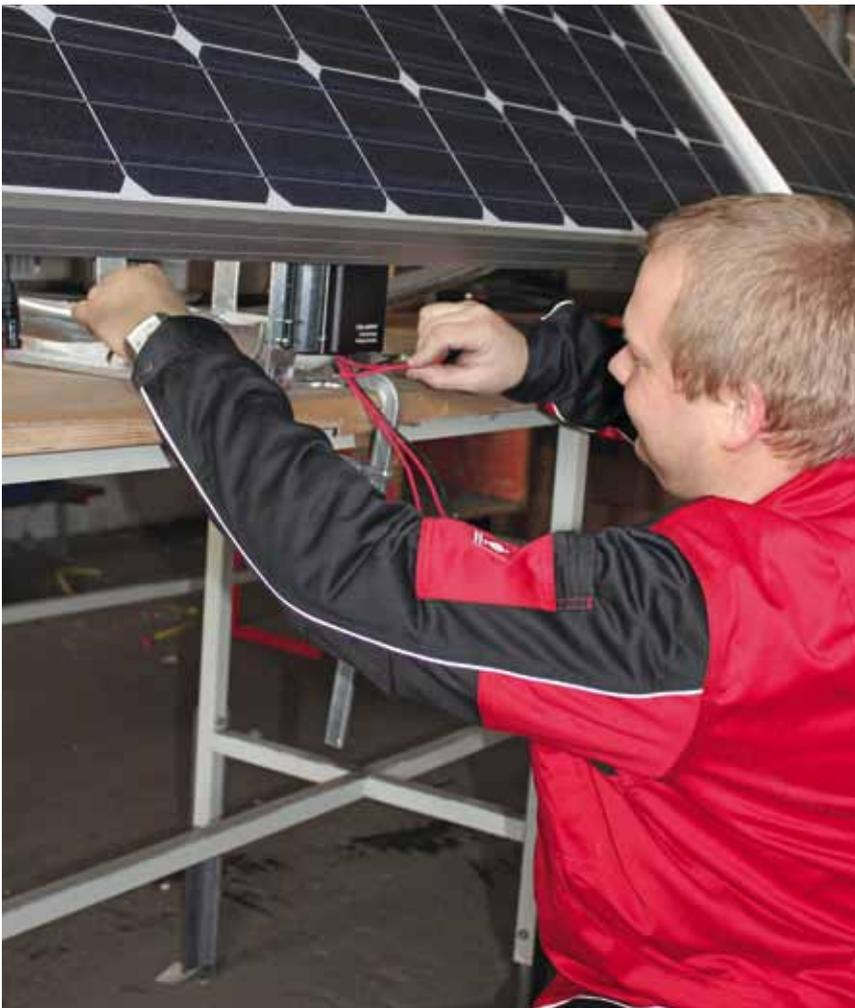
A Candilux technician installs the CIS-MPPT charge controller from Phocos with the Candilux solar module. Solar lights were installed along the access road to the sports field in Dellmensingen, a district of Erbach.
