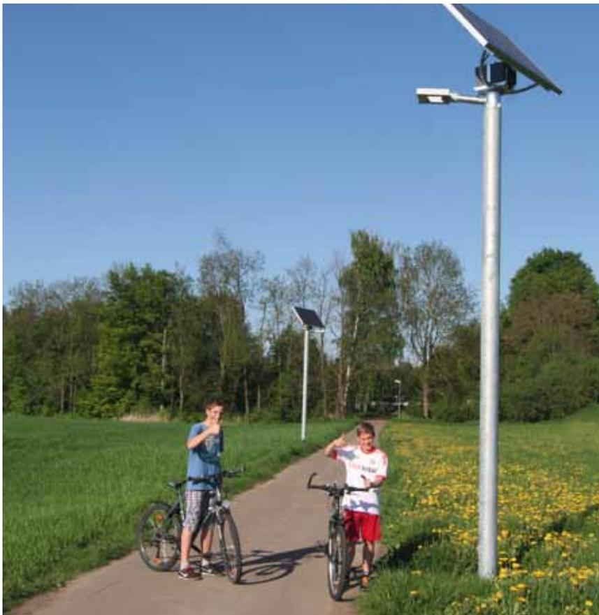
The CIS-MPPT charge controller from Phocos regulates the charging current and allows customized lighting settings. Thanks to the electrical charging unit and bright radiance of the LED lamps from Candilux, the solar lamps provide reliable light, even in the dark months of winter.
