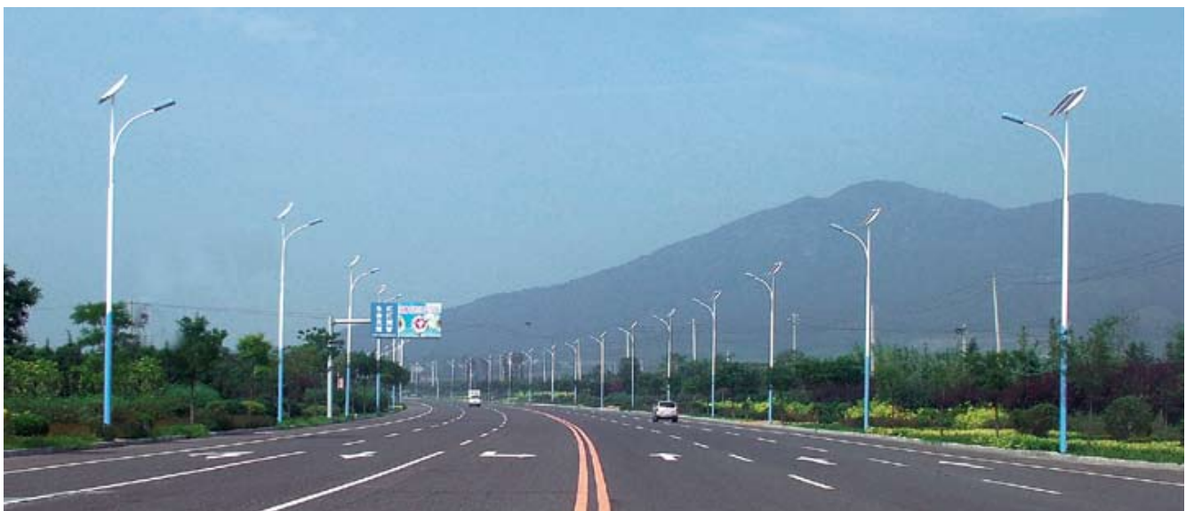
This off-grid street light application on Jimo Heshan Road, Qingdao, uses Phocos' fully encapsulated CIS charge controllers.
